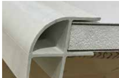
Fiberglass strands are woven together and PULLED through a die at high temp and pressure.
